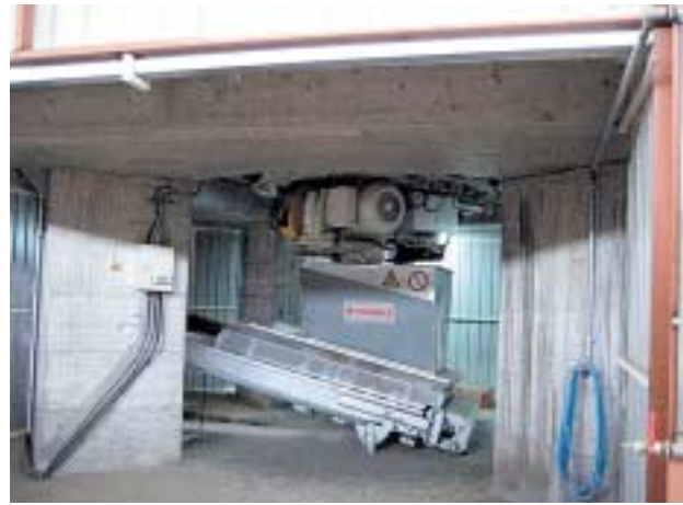
»11 Substructure of the clay silo, with auger feeding device
